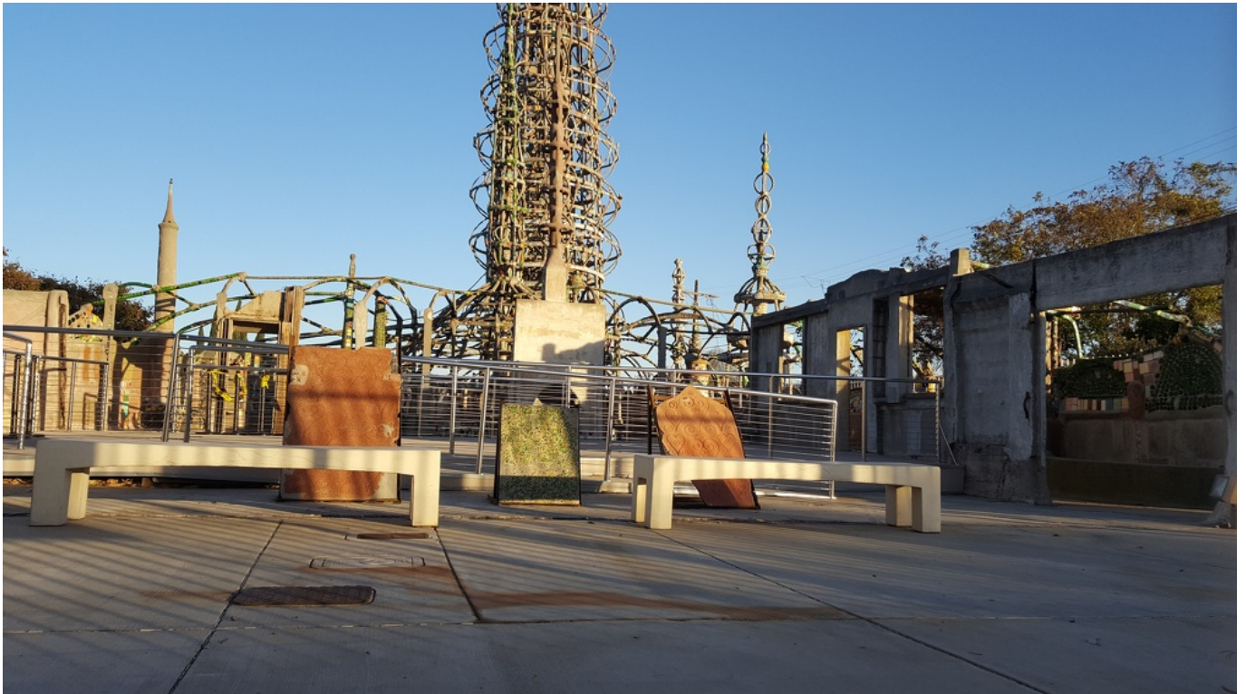
The off-limits-to-me base of the towers.
