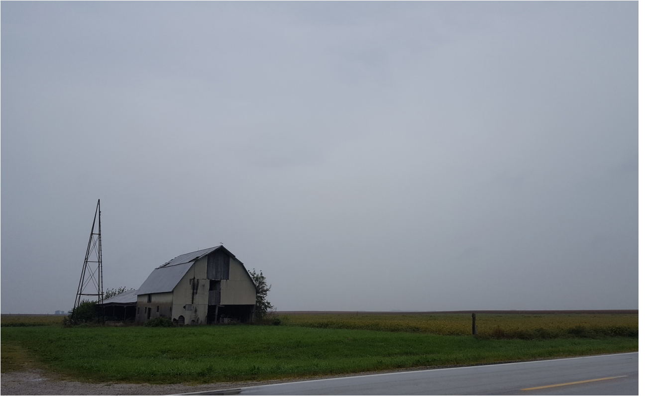
Run down rainy barn in Illinois II.
