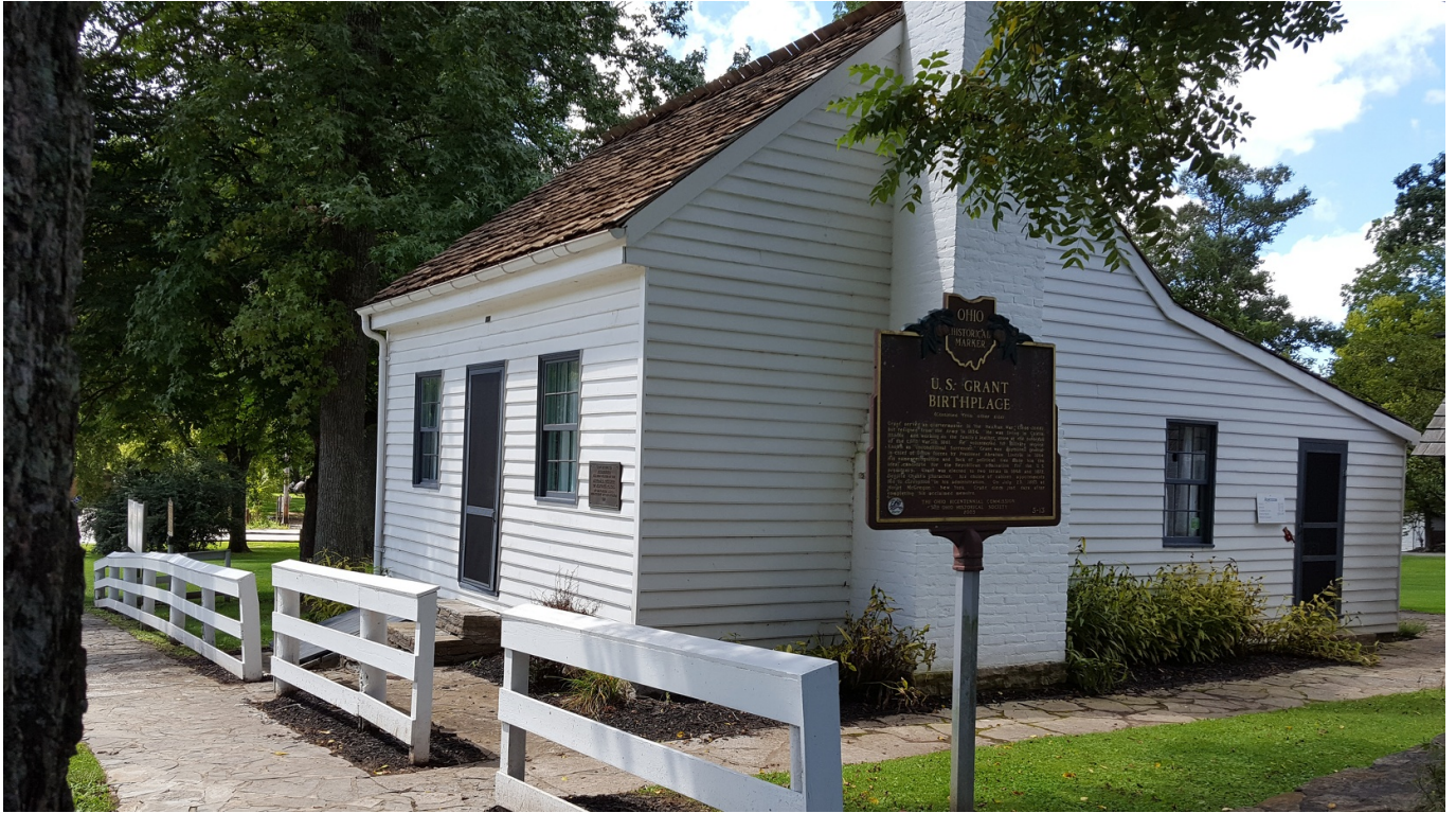
U.S. Grant Birthplace (building moved from nearby actual birthplace)
